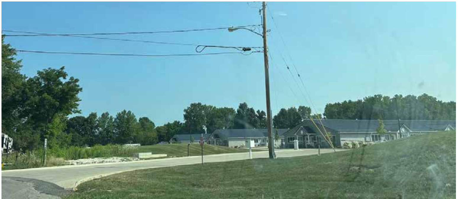
Figure 1. H-2A Worker Housing in Norwalk, Ohio
